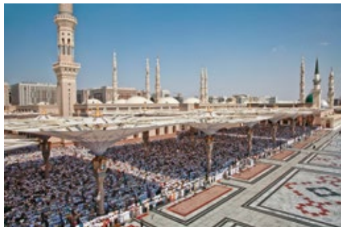
SL Rasch GmbH Special & Lightweight Structures, Madinah Piazza Shading Project, 2011, Medina, Arabia Saudita / Saudi Arabia, Courtesy SL Rasch GmbH | Special & Lightweight Structures
